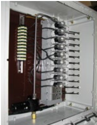
Instrument Box Fabrication
