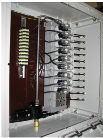
Instrument Box Fabrication
