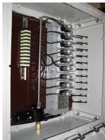
Instrument Box Fabrication
