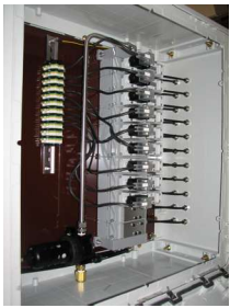
Instrument Box Fabrication
